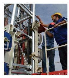
3. 免调试--防松滚轮和背轮:背轮滚轮调试完成后进行锁定,永久防松,用户直接安装,不用调试; No debug: Prevent loosing back wheel and idler wheel, locking back wheel and idler wheel after debugging
